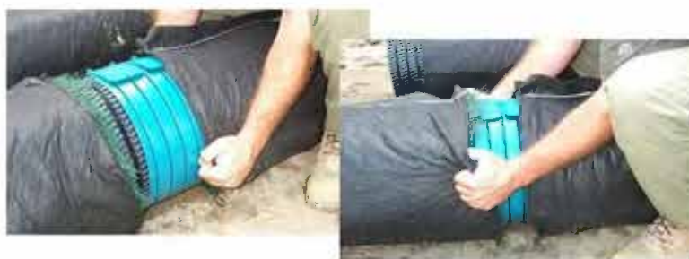
Figure 39. Replacing the geotextile over the couplings
