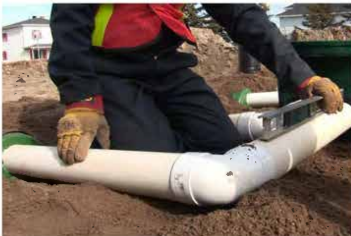
Figure 48. Inlet Pipe sloped toward Advanced Enviro-Septic
