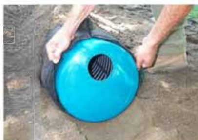
Figure 43. Installation of the Single Offset Adapter
