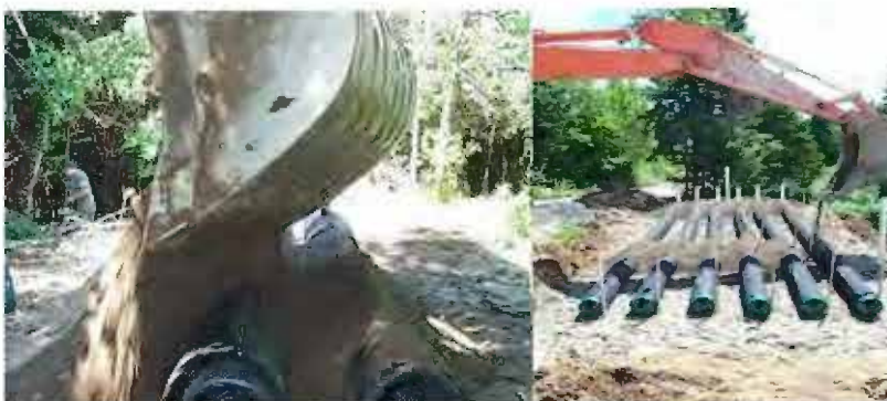
Figure 40. Covering the AES pipes
