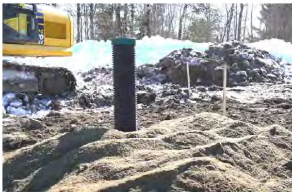
Figure 36. Final installation of the sampling device
