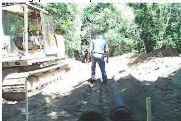
Figure 41. Filling the void around the Advanced Enviro-Septic pipes
