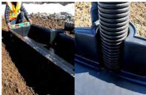
Figure 35. Sampling well installation
