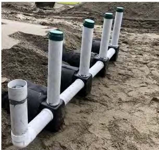
Figure 45. Entry vent on an extremity row
