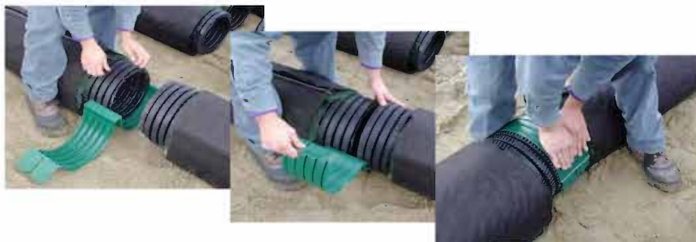
Figure 38. Installation of the couplings
